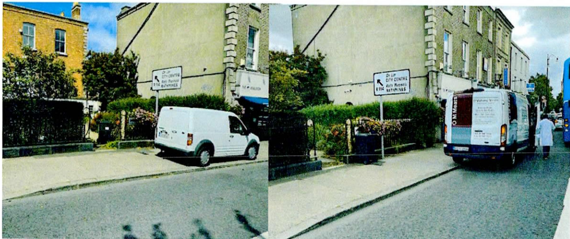
Figure 7.0 Imagery of the proposed bus stop location at No. 12 Terenure Road East – a protected structure. The bus stop is to be located in front of the original protected railings blocked by vans in the image above in an area used by the village shops for deliveries (as evident above and discussed further within).
